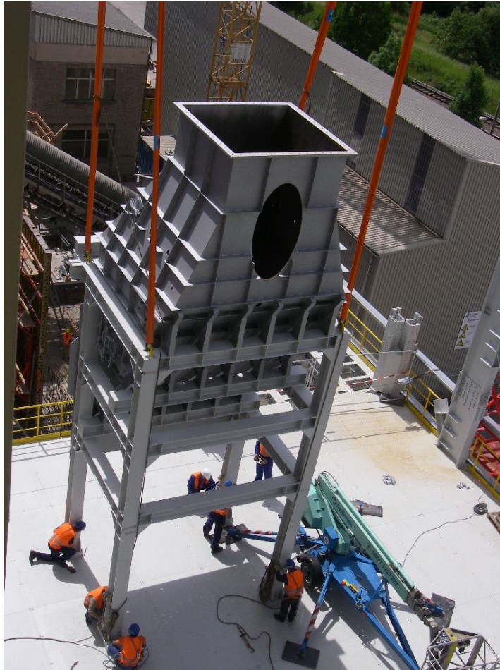
Kiln Inlet chamber
