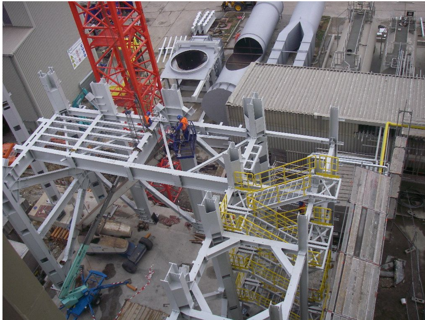
First beams of new preheater ins talled
