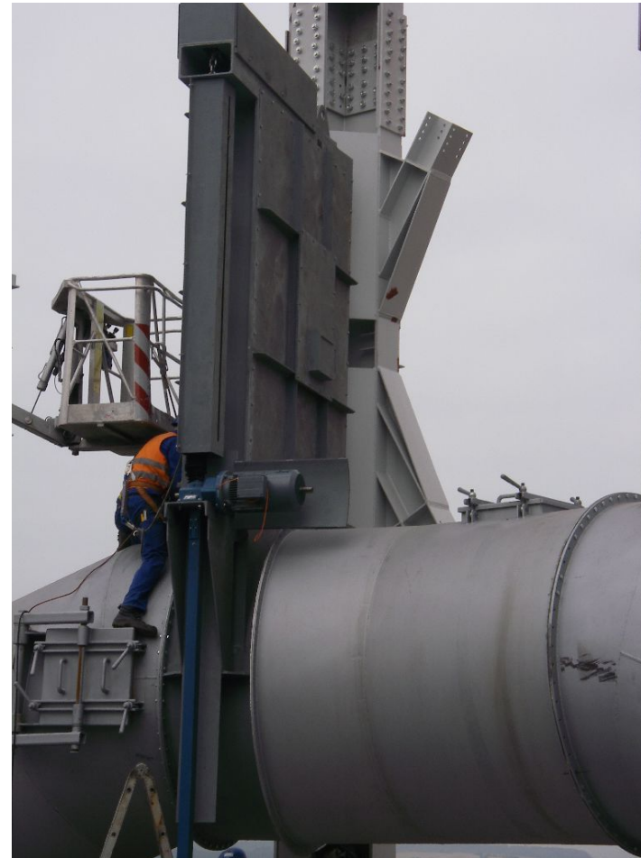
Tertiary Air Damper
