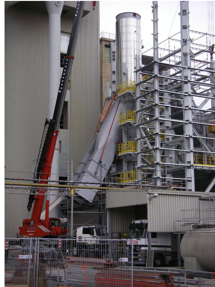
Hot Gas duct
