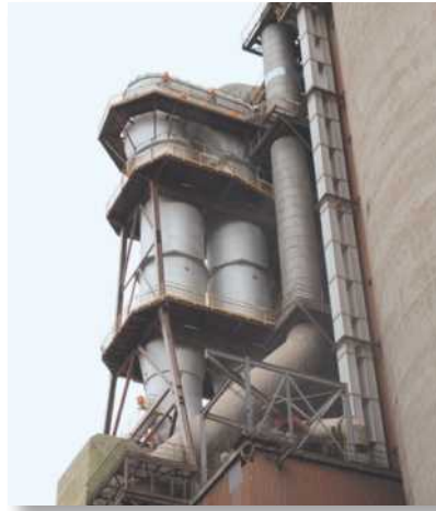
Figure 6: Calciner loop with the post combustion chamber in the Hranice kiln line
