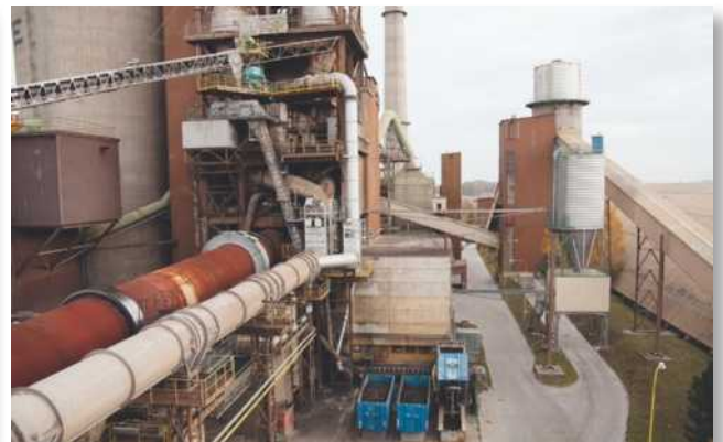
Figure 9: Photo of the DeNOx and hot gas chamber
