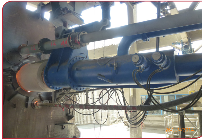
Right: A POLFLAME and separate injection pipe in a German cement plant.
