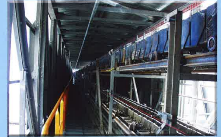
Clinker pan conveyor
