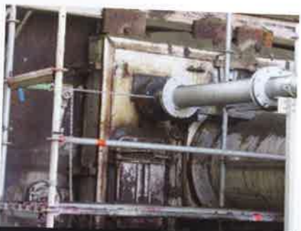
Figure 1: solid alternative fuel pipe in the kiln hood
