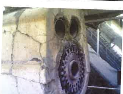
Figure 2: solid alternative fuel pipe in the burner refractory lining
