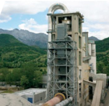
CEMENTIZILLO, Fanna Cement Plant
